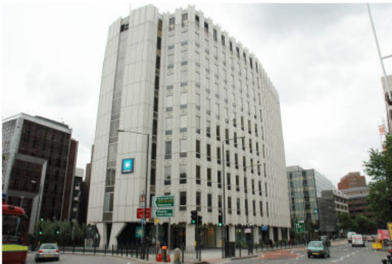
Existing building – taken from the Design and Access Statement
